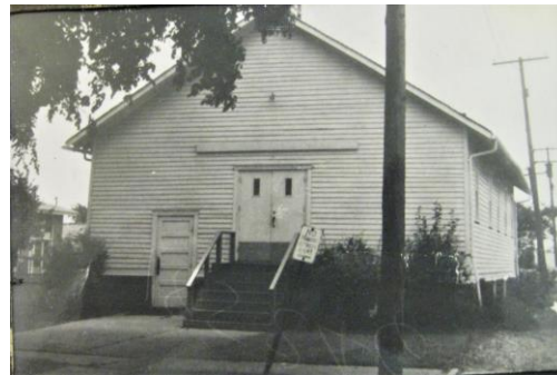
First Methodist Church Victoria Ave. (1921)
